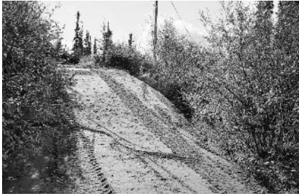
The City Public Works Department built a trail access ramp off the highway at the Mary Lake subdivision.
