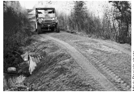
A new culvert is installed on the trail.
