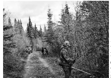
A KSA crew brushes the Mount McIntyre Road.
